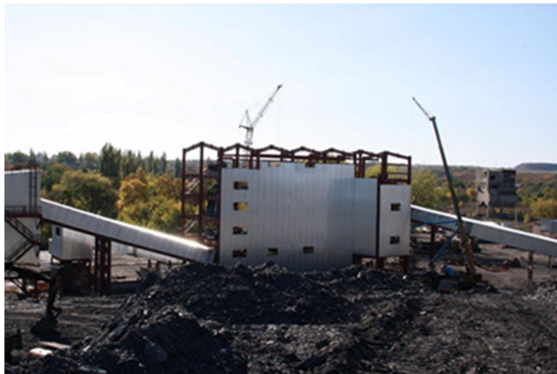
New processing plant construction progress
